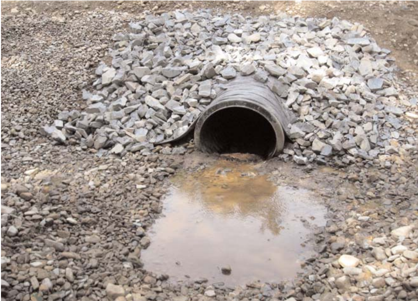
Properly installed cross-drain culvert (Photo courtesy of AV group)
