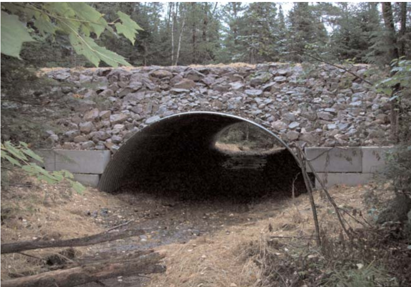
Top - Steel stringer bridge with bolt-a-bin abutments. (Photo courtesy of Fornebu Lumber) Bottom - Multi-plate open bottom arch. (Photo courtesy of AV group)
