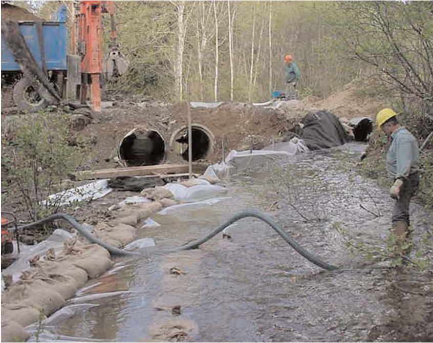
Stream Diversion with a cofferdam (Photo courtesy of AV Group)
